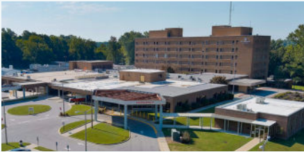
ECU Health North Hospital Roanoke Rapids
